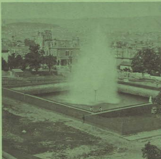
First Reservoir, Scranton Gas & Water Co. Corner Madison Ave. and Olive St.
